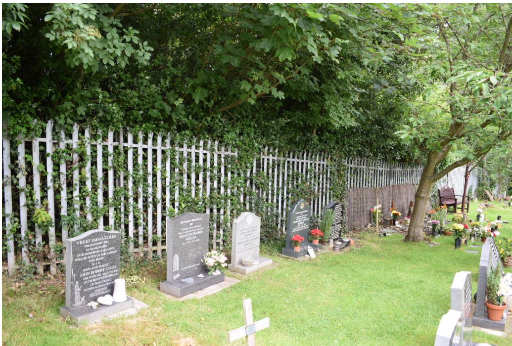
Figure 2: Palisade fencing along the rear boundary of the churchyard
