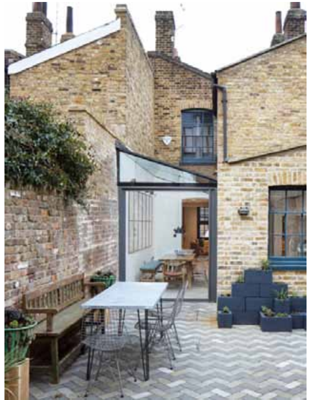
Side extension set back from established building line and using contrasting materials (Fraher Architects, London)
